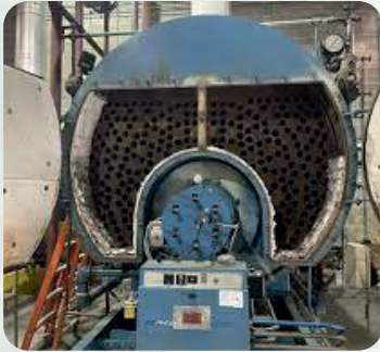
Boiler Repair & Maintenance Works
