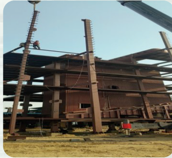
Boiler Erection
